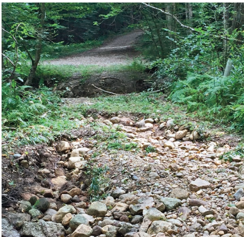
Washout at culvert on Falls Road over Tully Brook.
