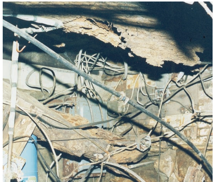
Plumbing and electrical panel under the Northeast chamber. The old floor joists completely rotted out. Wiring was still hot!
